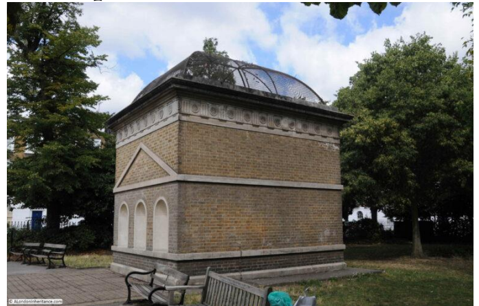
Victoria Line ventilation shaft in Gibson Square
