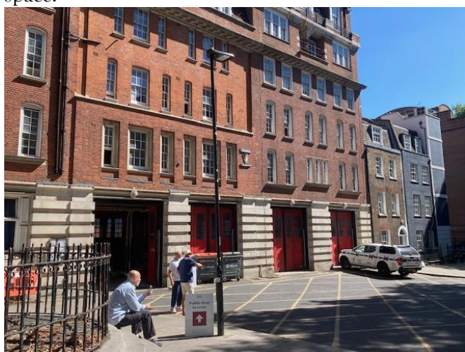
Clerkenwell Fire Station
