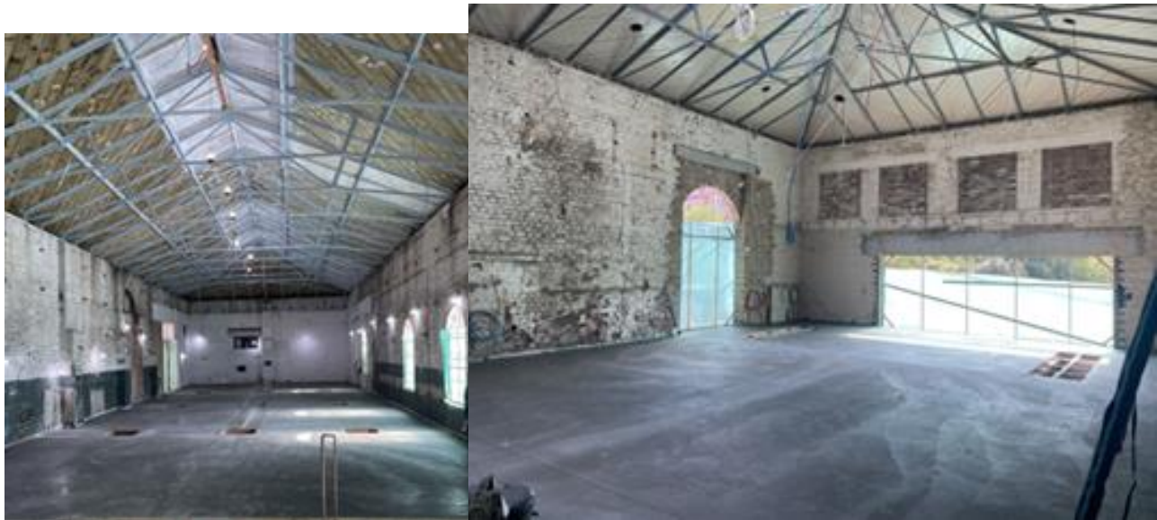
Left: the former Coal Stores which will become the largest of the three exhibition galleries; right: the Boiler House which will become the new café.
