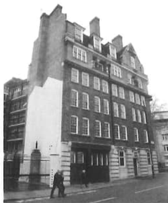
Clerkenwell Fire Station: doors are designed for horse-drawn and handcart fire engines
