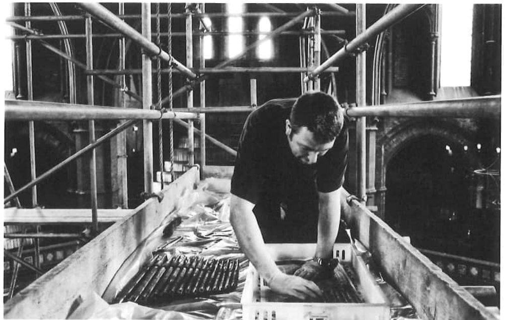
Above: organ pipes are packed up; below: Harrison & Harrison's restoration team
