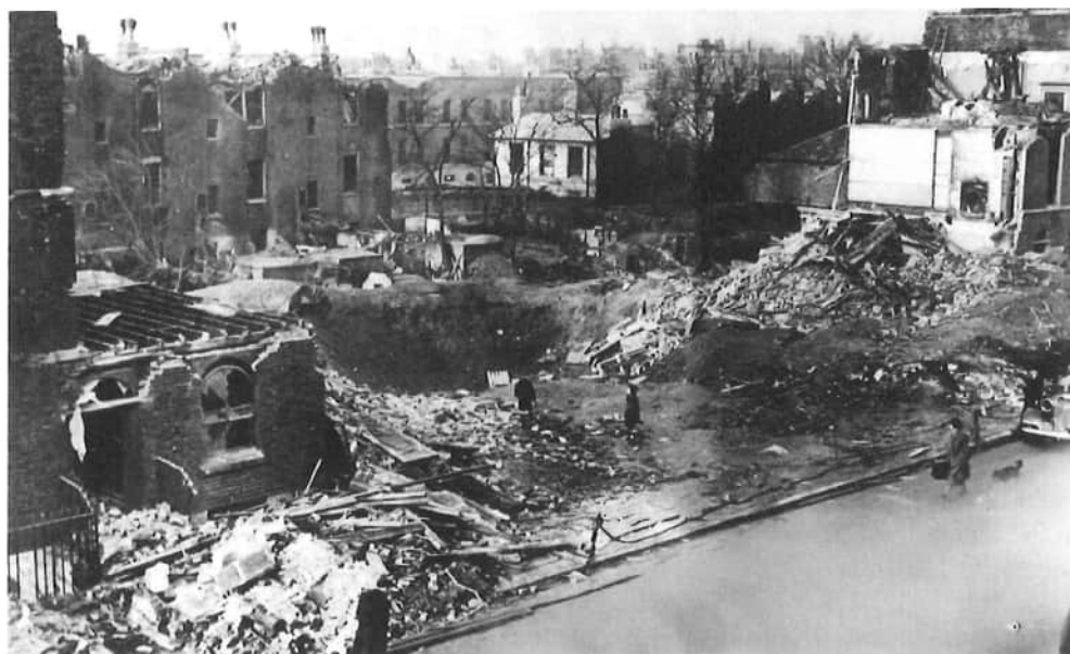
Bomb damage at Barnsbury Road, which crosses Copenhagen Street, in 1940
