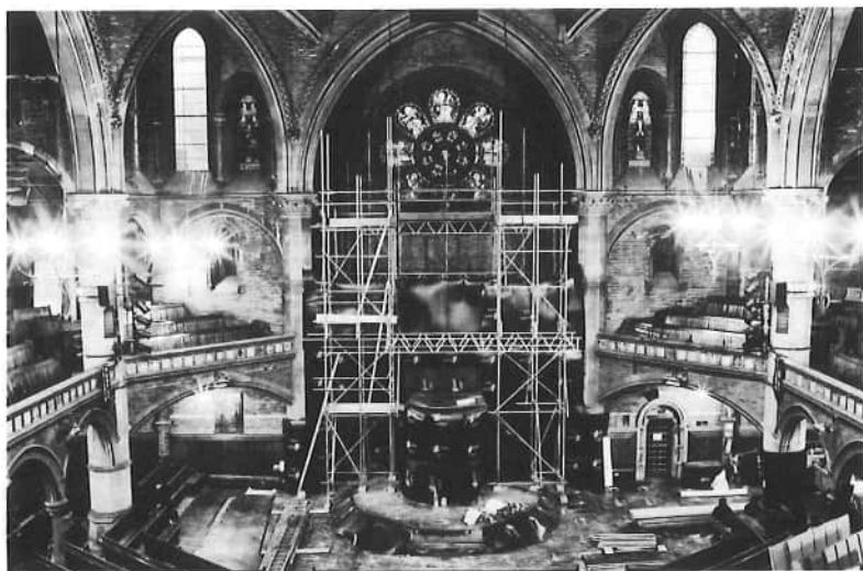
Removing the organ: the stage was taken down, scaffolding put up, and covers protected the pews and pulpit
