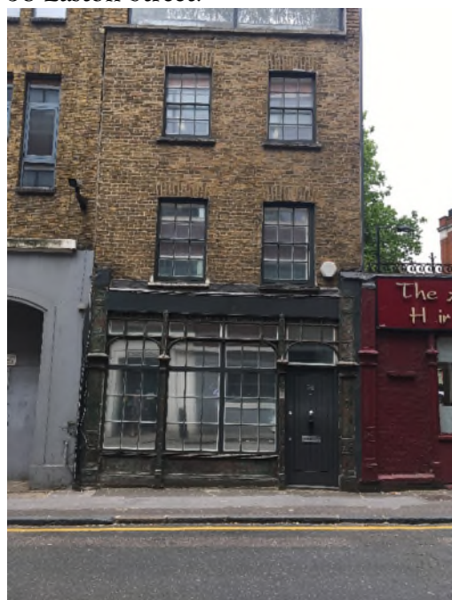
No. 38 Easton Street
