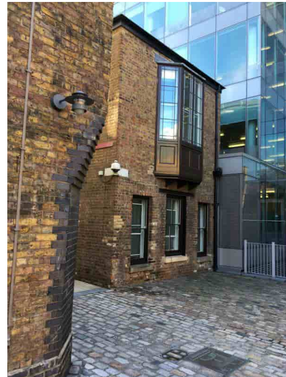
Albion Yard interior
