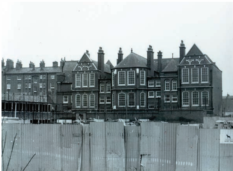
Charles Lamb Primary School: view from south-east, 1972
