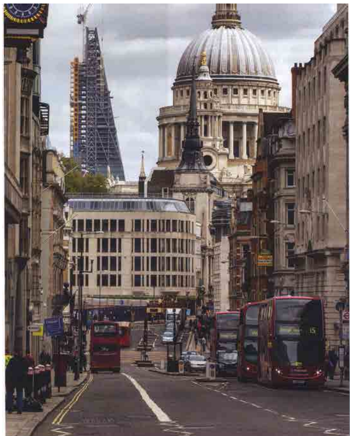
Respect for its context – the building's form tapers to fit with view corridors
