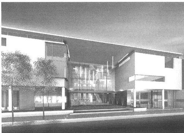
An impression of the new library at Finsbury Park.
