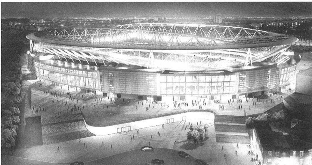
Everything around it has been altered but the sparkling stadium remains the same
